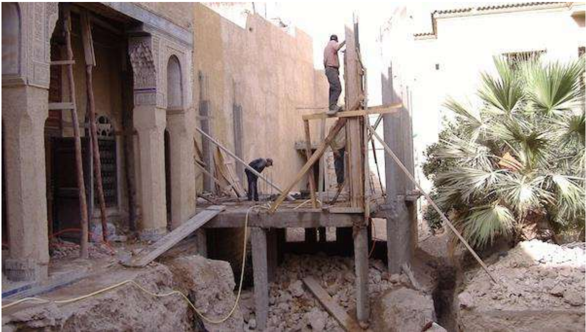
Stabilisation of the building's east wing.
