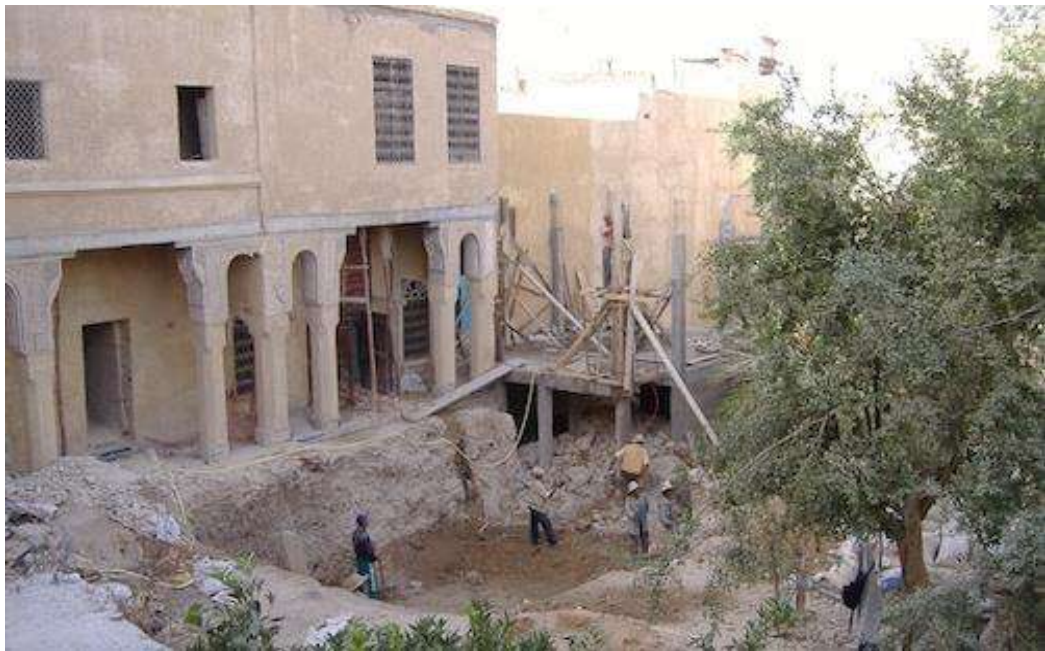
Excavation of the cellar and machine room
