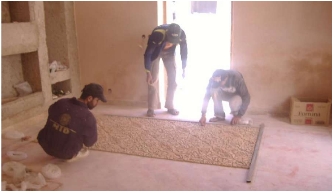
Zlejji in action. Here assembling the mosaics for the Odalisque restaurant. This work is done face down.
