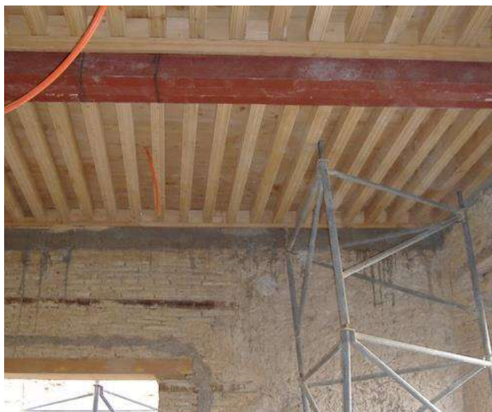
2008 – ceiling supported by steel I-beams in today's Suite Palmyre. Throughout the house, all cedar ceilings had to be completely done new.
